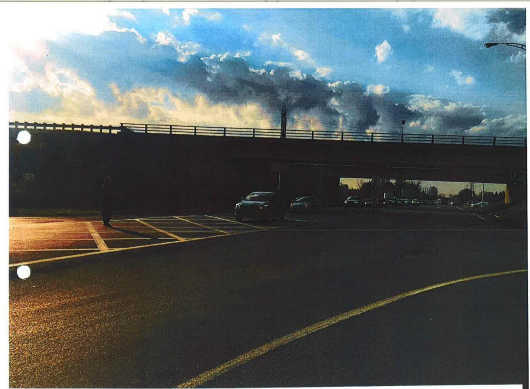
(3a) P.K. TRAFFIC CONTROL HWY.30/207 INTERSECTION - (Sept.20/16 - 8:25 a.m.)
